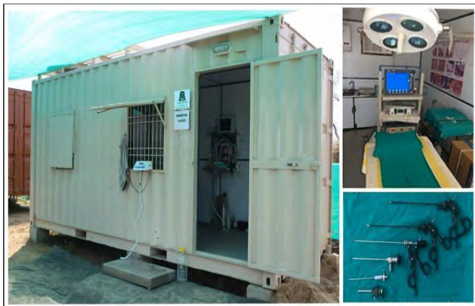
Fig 3: Customized operation theatre facility along with laparoscopic unit and instruments
